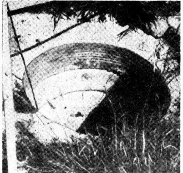
The mouth of the well. It is intended to build up the wall above ground level and fit a cover.
